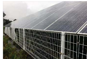
(不適切な柵塀設置の事例)
