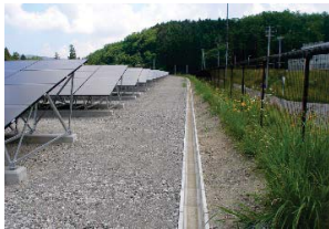
(適切な柵塀設置の事例)
