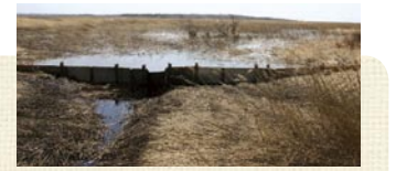
Banks to prevent the lowering of the wetland water level
