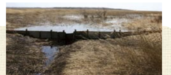
Banks to prevent the lowering of the wetland water level
